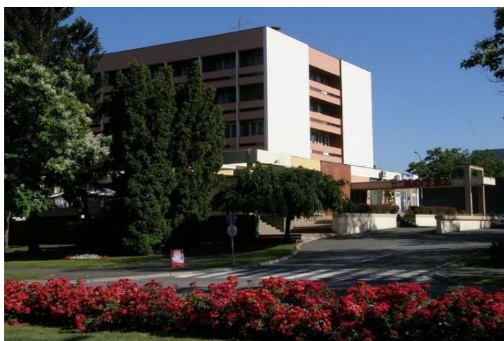
Slika 9. Hotel Kalnik ( https://krizevci.hr/adresar/hotel-kalnik/ )
